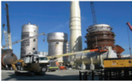
Installation of Alloy Towers
