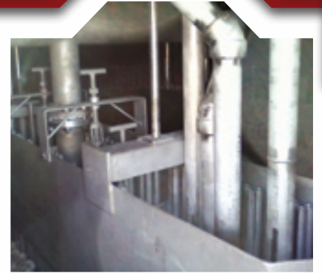
ZeCor UniFlo distribution troughs for the interpass tower.
