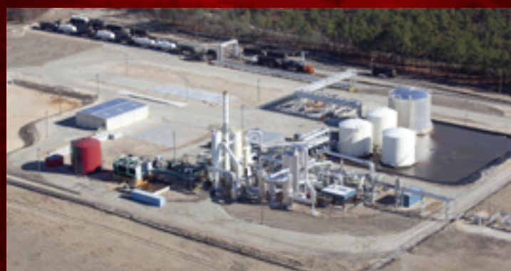
Southern States Chemical, Inc.'s new state-of-the-art Wilbara sulfuric acid plant in Wilmington, N.C.
