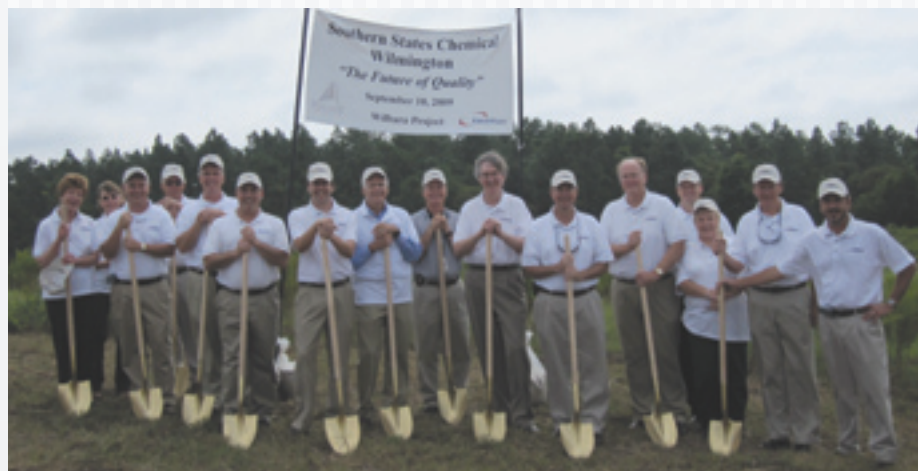
At the September 2009 groundbreaking, many were on hand to start construction of the new plant, which began operation in December 2010.
