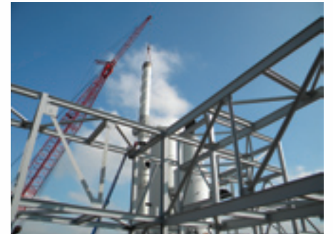
Topping off the stack at the new facility.
