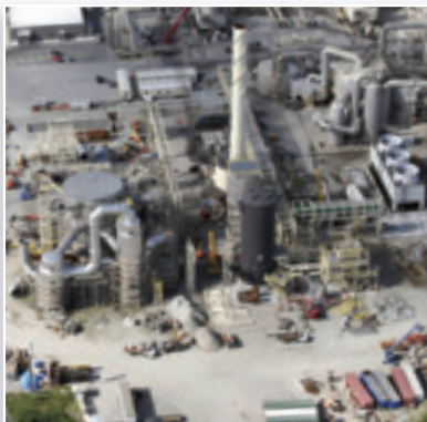
Plant at 50% status with completed alloy towers
