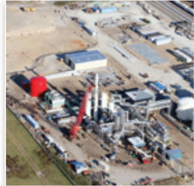
Greenfield sulfuric acid plant fabricated & constructed, Nov. 2010
