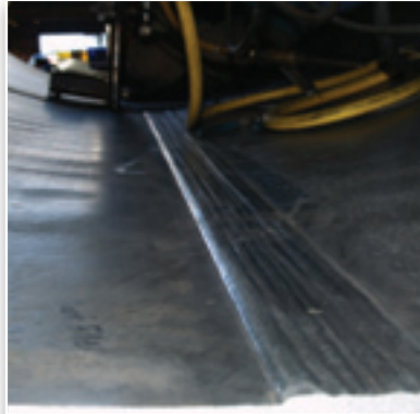
Overlay clad nickel alloy cover pass for duplex reactor
