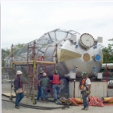
Equipment job site insulation and stairway installation
