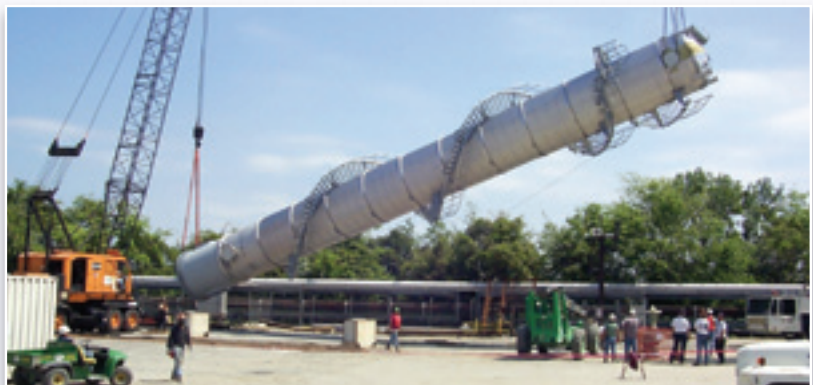
Lift plans, heavy rigging, and equipment installation
