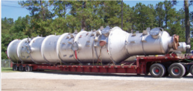
Top section of fabricated 10' diameter x 200' tall 904L column delivered to the job site
